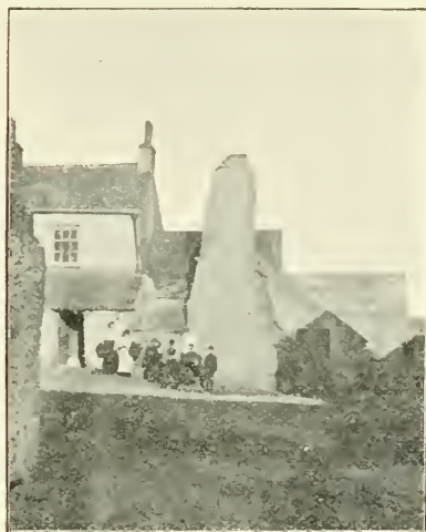
OLD CHIMNEY AT PHILBEACH. From a Photo. by F. Green.
